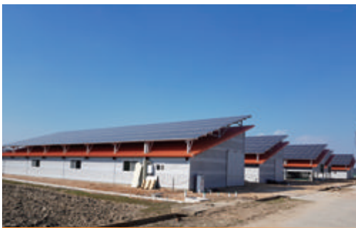
Project Size: 640KW Installation Site: Korea
